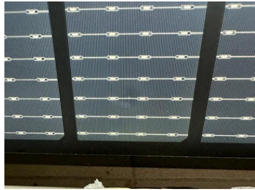
Figure 6.32: Category C Defect
