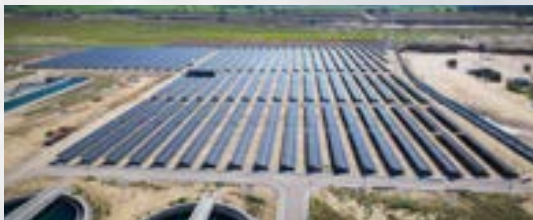
Gaza Central Wastewater Project
