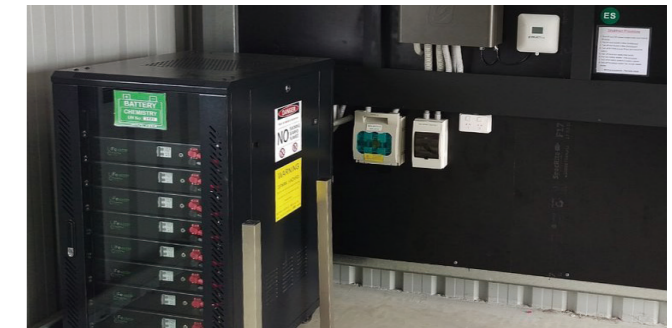
Rack-mounted lithium battery
