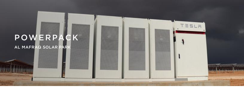
"The new power plant's purpose is to enhance the grid by power peak shaving and power shifting to increase the stability of the grid and support the grid at peak load hours. Additionally, it will also enhance the availability of energy during daytime hours and the remaining Energy to support the grid during nighttime Hours." Philadelphia Solar
